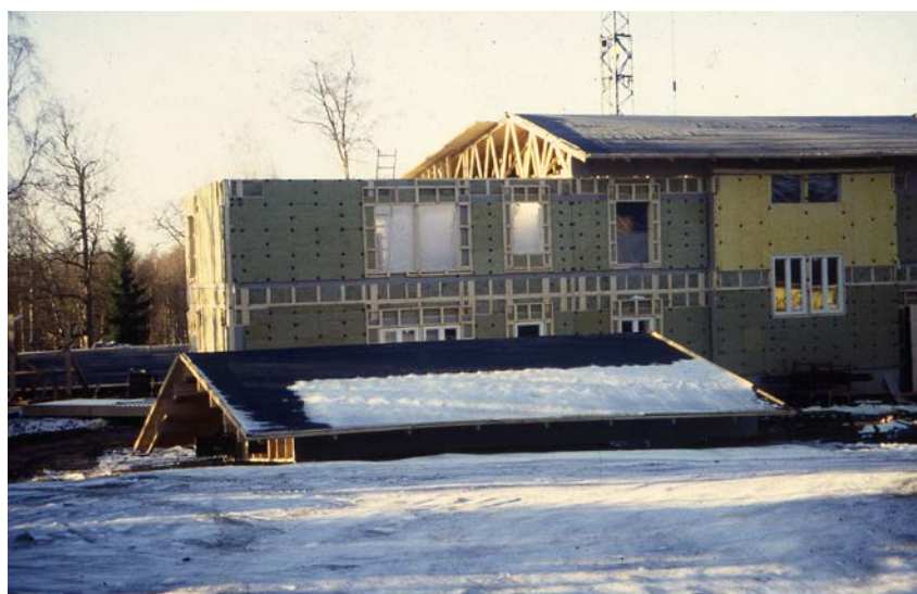
Figure 8.13: Roof used as weather protection during erection of the structure.
